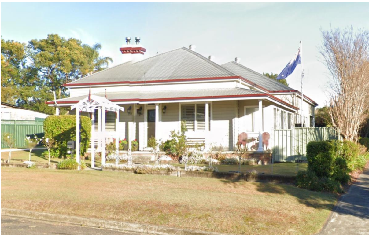
Figure 5: Photo of 58 Lord Street with the existing weather board dwelling shown
